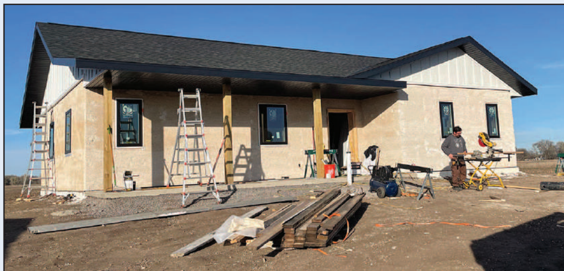
A 4-bedroom hempcrete house being built at the Lower Sioux community. The Lower Sioux Hemp and Housing Program is leading the way for Native communities to utilize hemp for sustainable, energy-efficient housing. (Photo by Ashley Satorius.)
